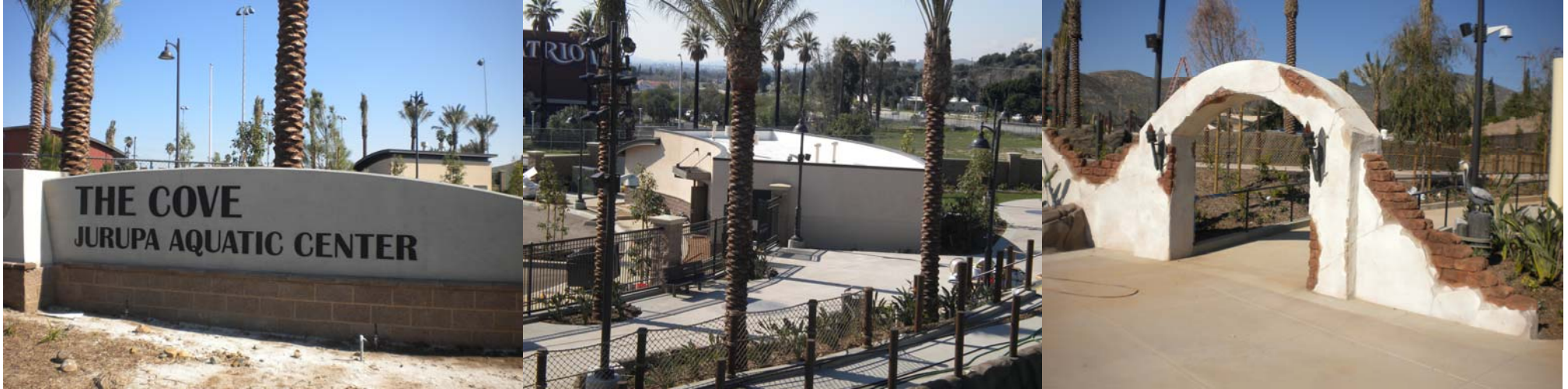
The Cove, Jurupa Aquatic Center – Riverside, CA
